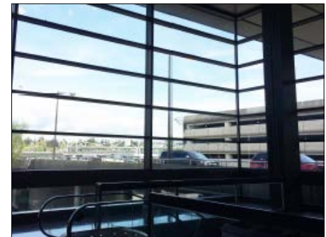
Shatter proofing (Phase I)
