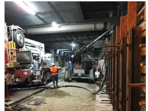
West Wall Seismic Reinforcement
