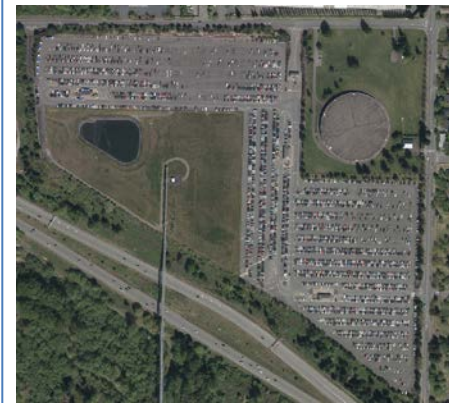
Existing NEPL Facility
