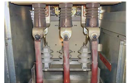
Shown here (before any cleanup) is the interior of switchgear that was protected by SEL light-sensing and overcurrent protection during a 6.6 kV arc-flash event. Damage was limited to arcing on the cable termination bolts.
