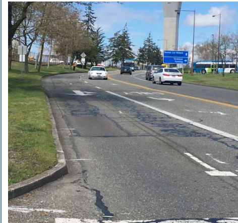
Existing Roadway Conditions
