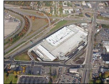
Consolidated Rental Car Facility
